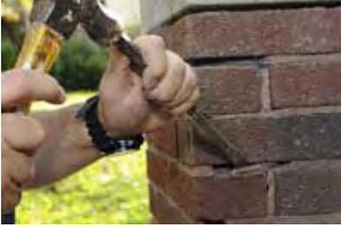
To remove deteriorated mortar properly, hand chiseling is the method least likely to cause damage to the
