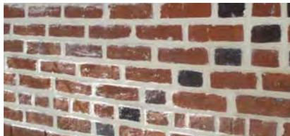
We recommend that the mason complete a test patch (a sample area of repointed joints). Once the test patch is inspected to determine that the masonry has
